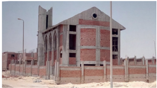
Church being built in New Assiut City
