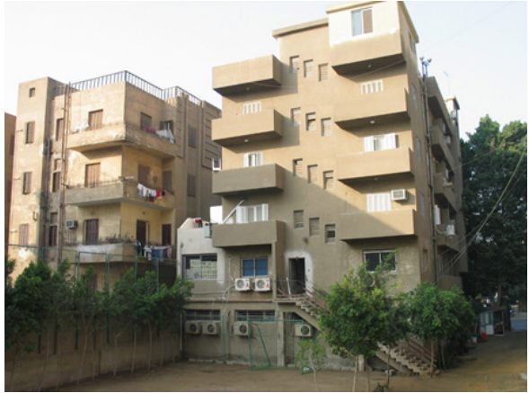
At left, property next to Evangelical Theological Seminary in Cairo, bought by a Christian businessman. The first floor was completely renovated for the seminary's expansion.
